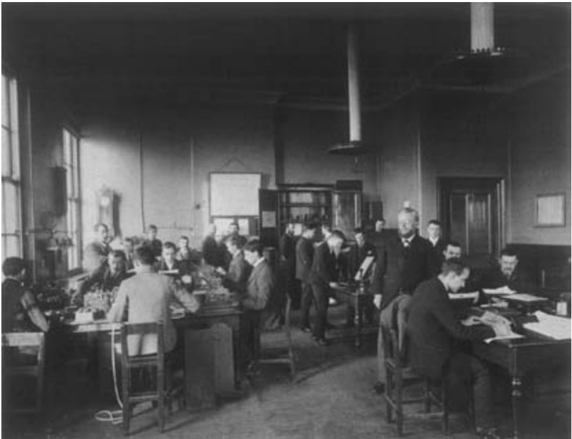
Figure 6 The Great Northern Telegraph Company's Newcastle office in the 1870s. The young men on the left are sending and receiving Morse-coded messages using Wheatstone's automatic apparatus, and the boys standing at the table are collecting telegrams for delivery. Courtesy of GN
